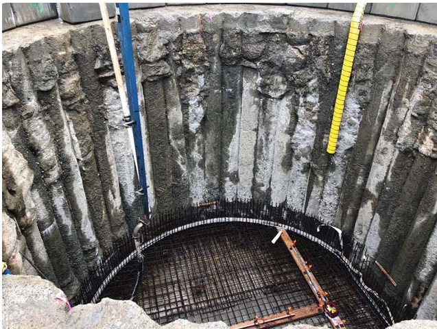
Raw Water Pump Station: Caisson/Tunnel Shaft - Base Slab Concrete Pour
