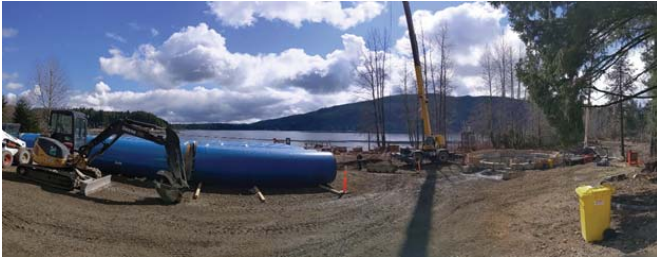
Raw Water Pump Station Site: Pipe ready to be tunnelled into the lake.
